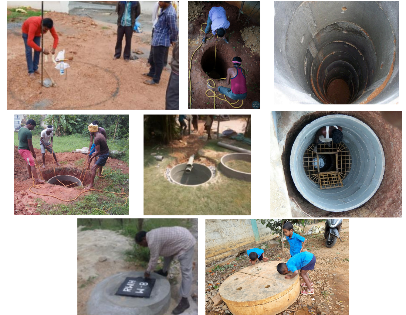
Figure 27: Images representing step-wise implementation of recharge wells.
